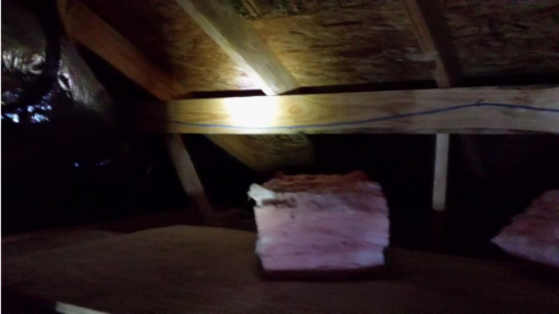
This section of knee wall has a 2x6 purlin.
